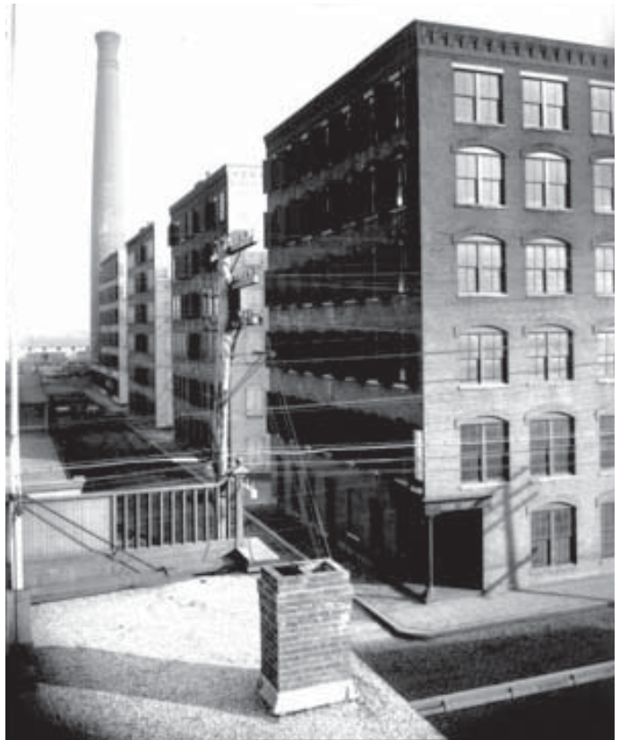
Wormwood Factory Building, 1898
