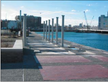
Harborwalk under Construction
