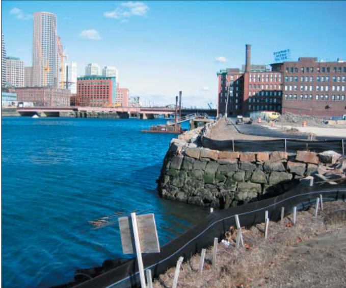
Harborwalk under construction along Gillette property, 2004
