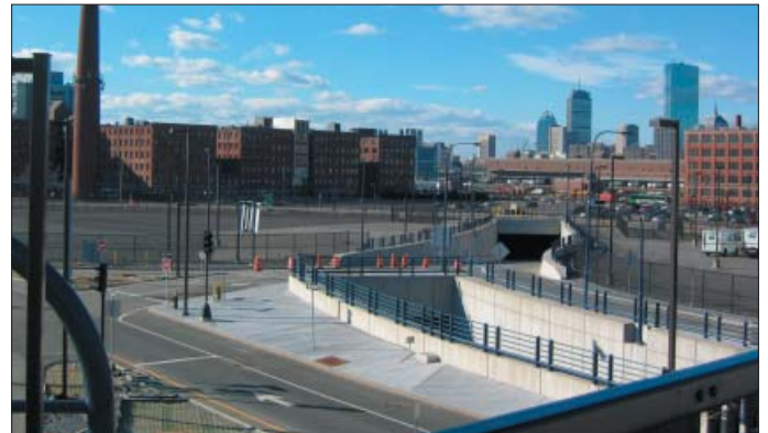
I-90 Exit Ramp at Haul Road and Summer Street
